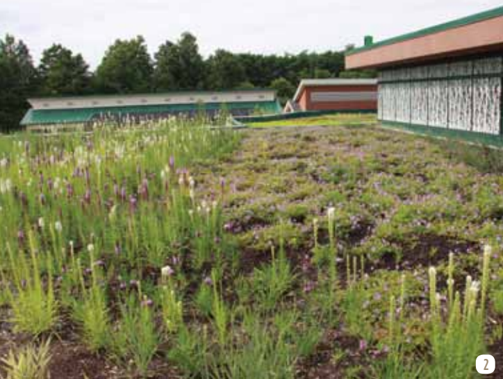
1,000 M 2 OF GREEN ROOF FEATURES 7.5-15 CM OF GROWING MEDIUM, AND MORE THAN JUST SEDUMS [2].
