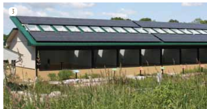
THE NATURALLY VENTILATED AND DAY LIT AVIARY FEATURES A 28KW PHOTOVOLTAIC ARRAY [3].
