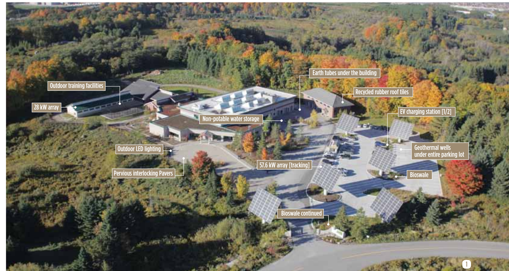
THE PROJECT SITE HAS FEATURES MANY ORIGINAL LOW-IMPACT DESIGN FEATURES AND UPDATES TO GENERATE AND CONSERVE ENERGY [1].
