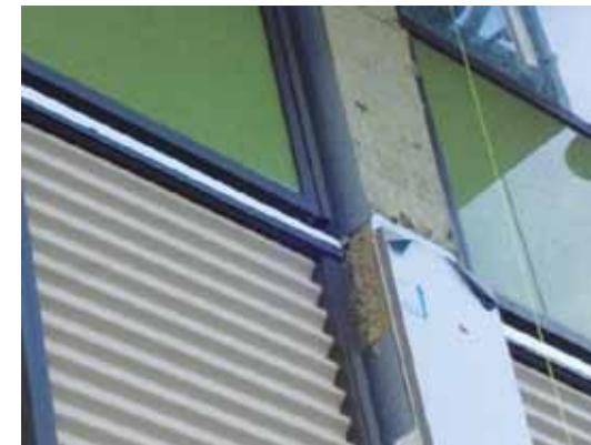
AN EXAMPLE WHERE THE ASSEMBLY U-VALUES MIGHT BE FINE WHEN THINKING IN PARALLEL, BUT THE OVERALL THERMAL PERFORMANCE IS POOR BECAUSE OF THERMAL BRIDGING AT INTERFACE DETAILS.
